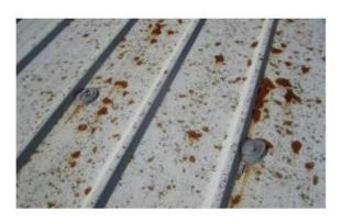
Figure 8 Cover fastener heads as needed
