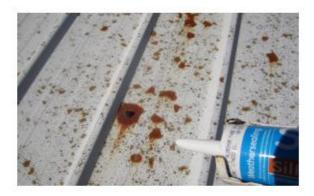
Figure 7 Fill small holes with sealant
