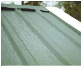
Figure 4 Silicone coated metal roof
