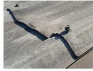
Figure 3 Corroding and Loose fasteners
