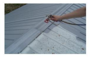
Figure 13 Coating of ridge cap
