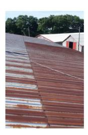
Figure 2 Corrosion can be either be Localized or Uniform
