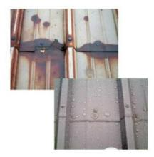
GE Enduris™ protects superficially rusted metal surfaces, renewing the roof system and extending its life span. Deeper or flaking rust on panels may need to be removed by wire brush, sandblasting or mechanical abrasion until all scaling is removed. Review the "surface preparation" section below for additional information.
