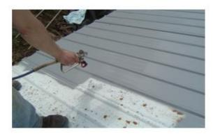
Figure 11 Panels being coated
